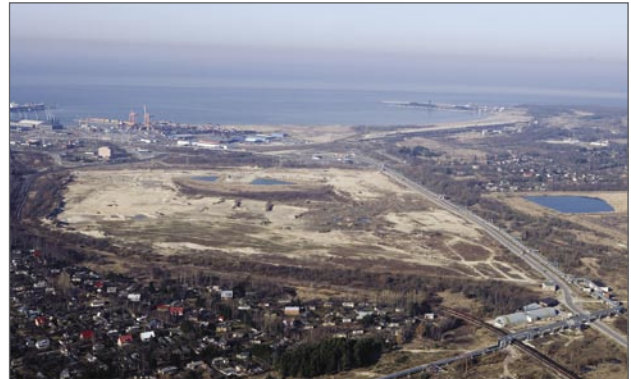
• Under development. New Corporate Park NordShore, Muuga Harbour.
